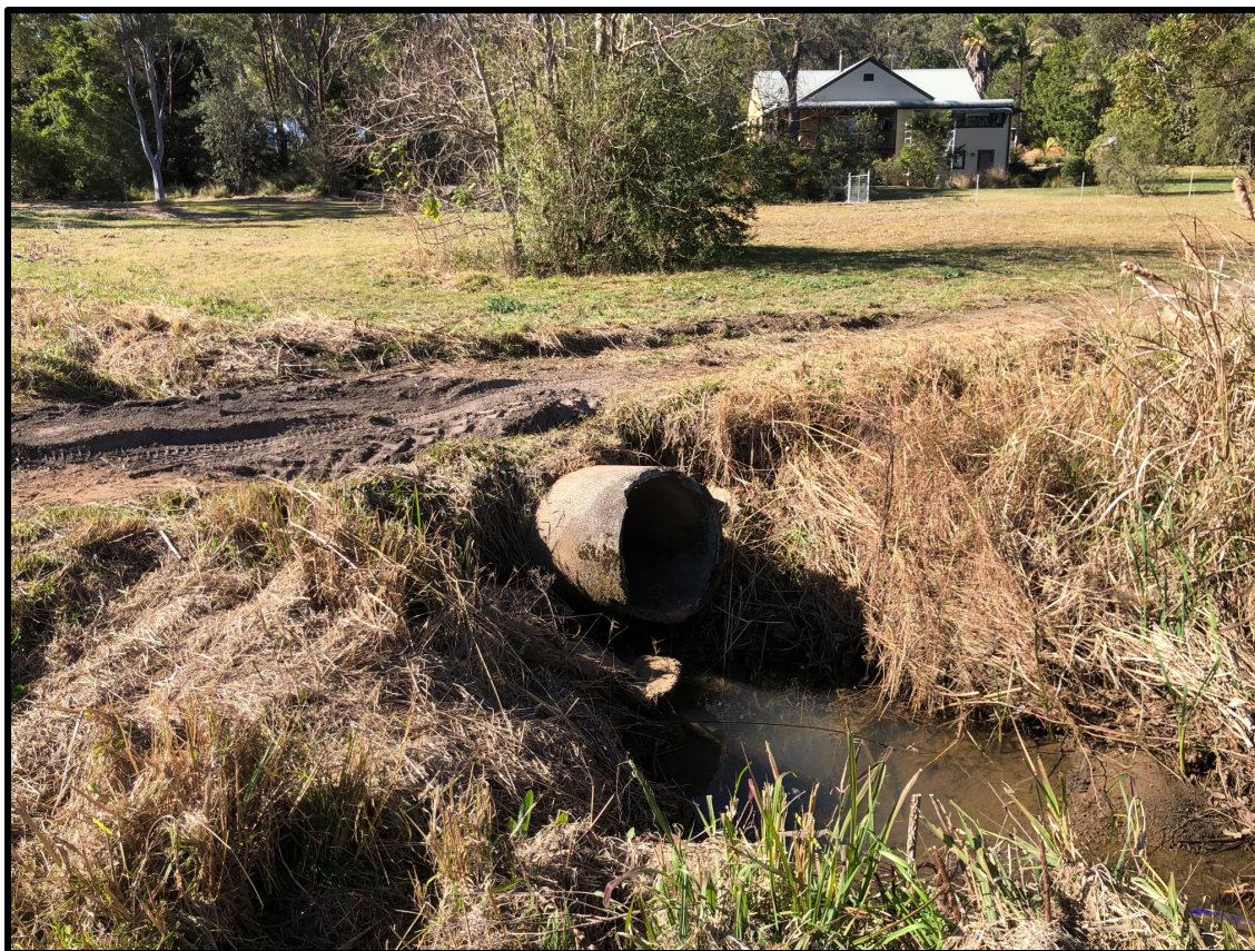
Figure 25. Cuvert and Dam at no 52 Ferodale Road.
